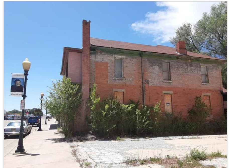
Vacant buildings in Raton
